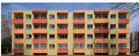
Ichinoya Residence Area
